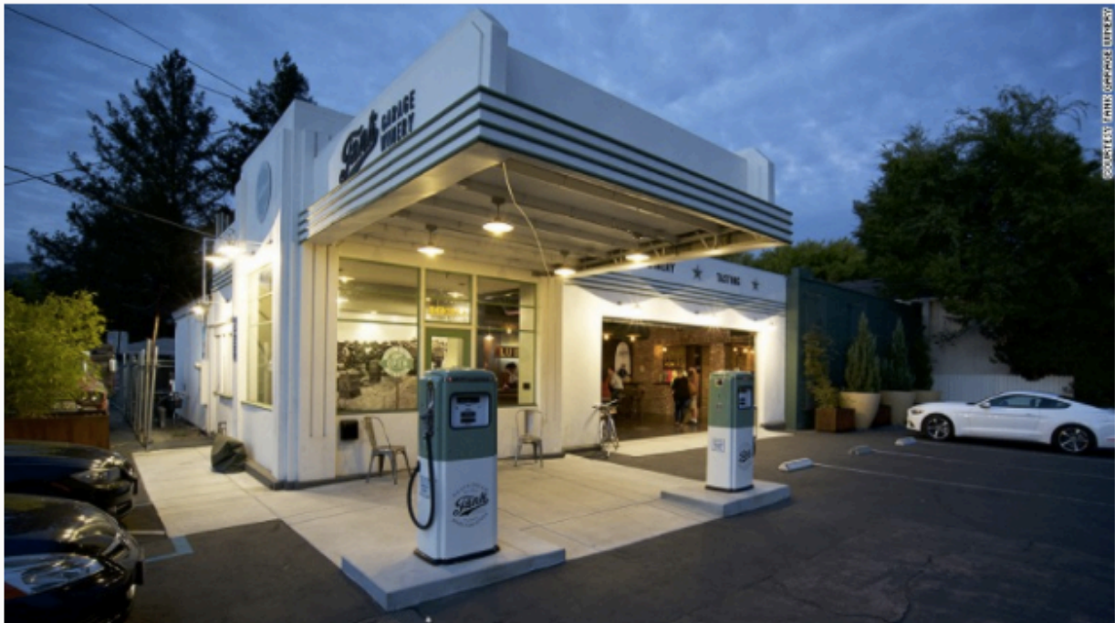
Tank Garage Winery: California Lubrication.
